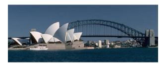
The construction of the Opera House is only possible because the distinctive shells come from a single geometric spherical section. This was not part of the napkin design — yet according to Utzon, this "solves all the problems of practical construction by opening up mass production" both for the tiles on the roof, and the ribs supporting them. Without mass production of modular components the Opera House could not have been completed.
